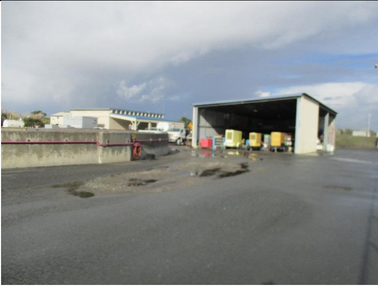
BEFORE: PAVEMENT AT NORTHEAST CORNER BY CARPORT
