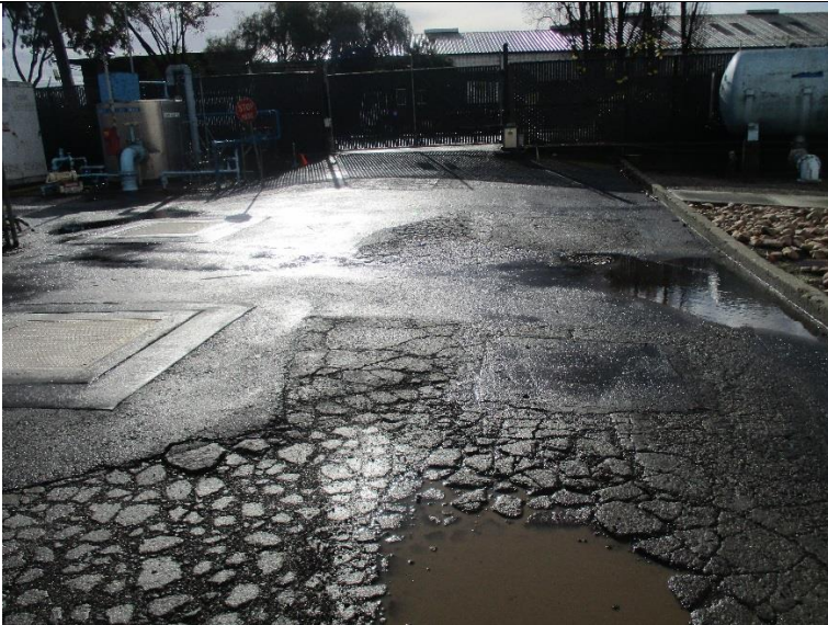
BEFORE: PAVEMENT AT DAVIS STREET SERVICE GATE
