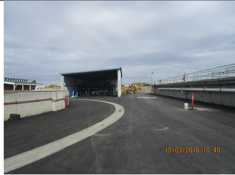
AFTER: PAVEMENT AND CONCRETE DRAINAGE SWALE AT NORTHEAST CORNER BY CARPORT
