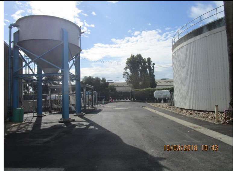
AFTER: PAVEMENT AND CONCRETE SWALE AT DAVIS STREET SERVICE GATE
